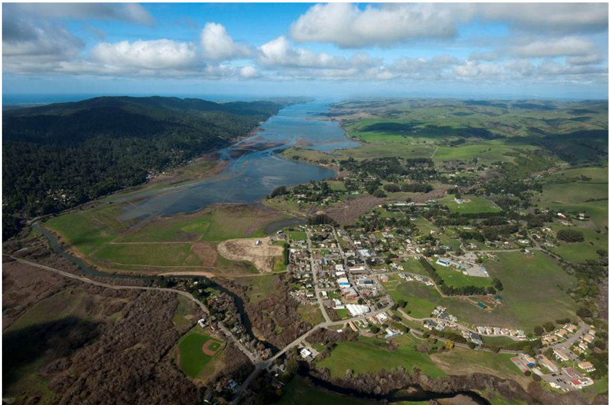
Giacomini Wetland following removal of the levees and reconnection of Tomasini Creek. Photo by Robert Campbell
